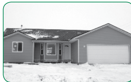
Ray High/View Housing Project in Ray, ND
